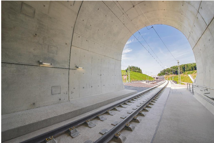
Caption picture 1: RHEDA 2000® installed in tunnel in Hanau-Nantenbach, Germany (picture: PCM RAIL.ONE AG)
